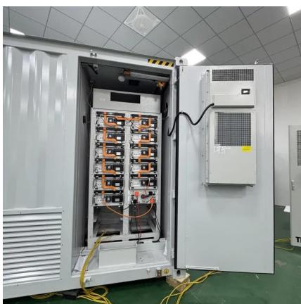
[200kwh Lithium Battery Energy Storage System Bess Solar Container](#)
